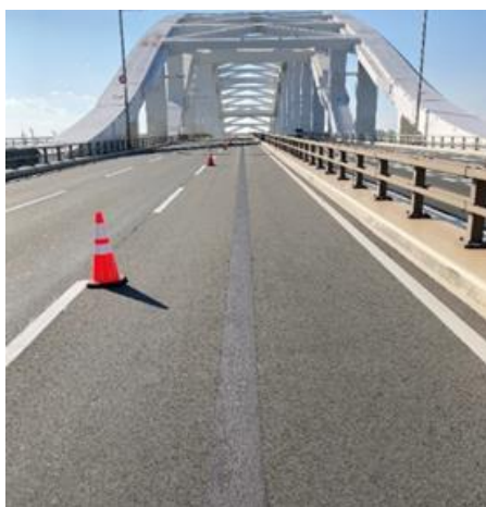
The Paint Can Be Customized in Colors That Visually Blend with the Road Surface
